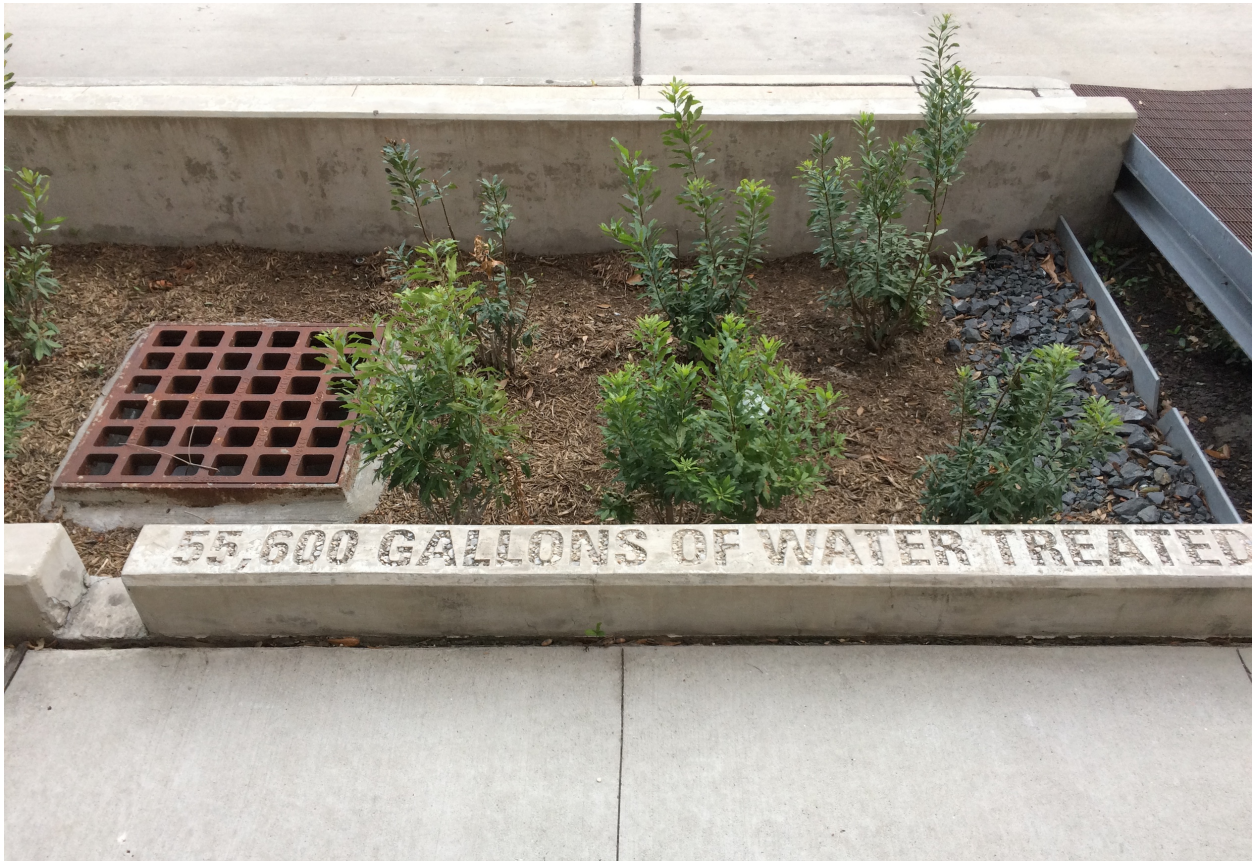
Cover: HEB Children's Rain Garden, Zach Scott Theater, Austin This page: Rain garden, Bagby Street, Houston
