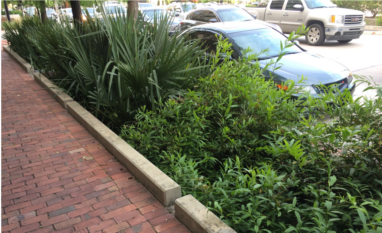
Permeable pavement and rain gardens, Bagby Street, Houston
