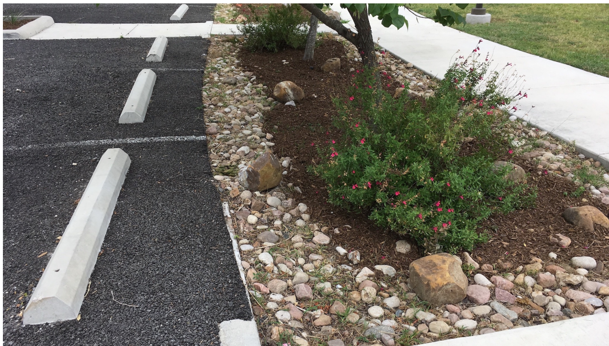
Permeable pavement and bioswales, Mission Branch Library, San Antonio
