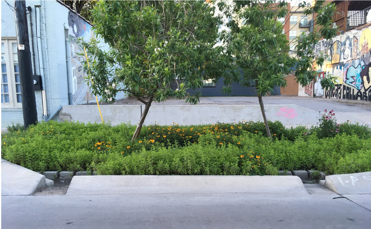
Rain gardens, Elm Street, Dallas
